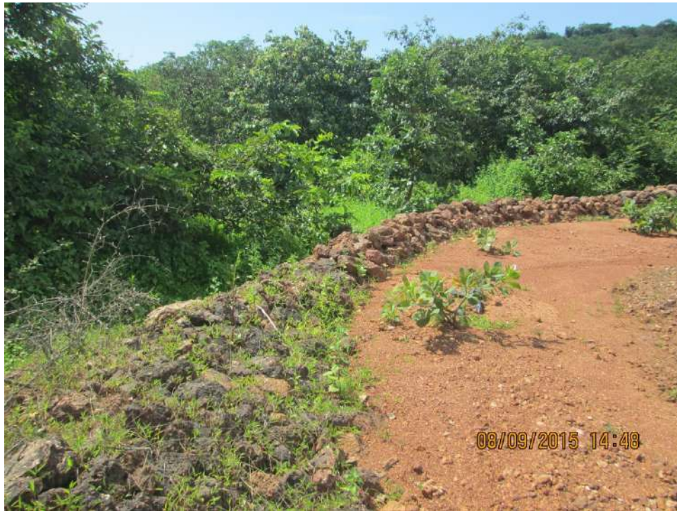
Retention Walls within lease area
