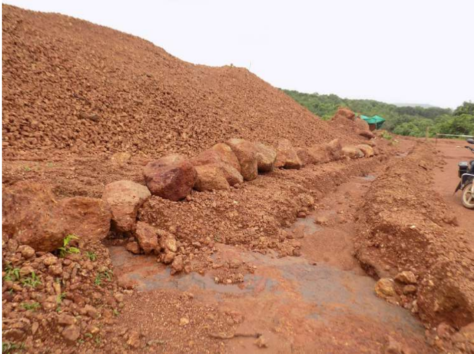
Drains to collect and channelize the rain water around bunds
